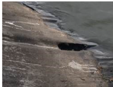
Tears in the Aging Lagoon Liner
