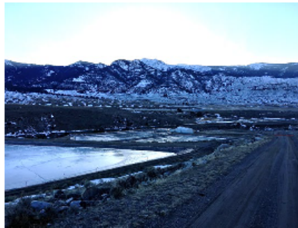
Gardiner Park County Wastewater Treatment Facility
